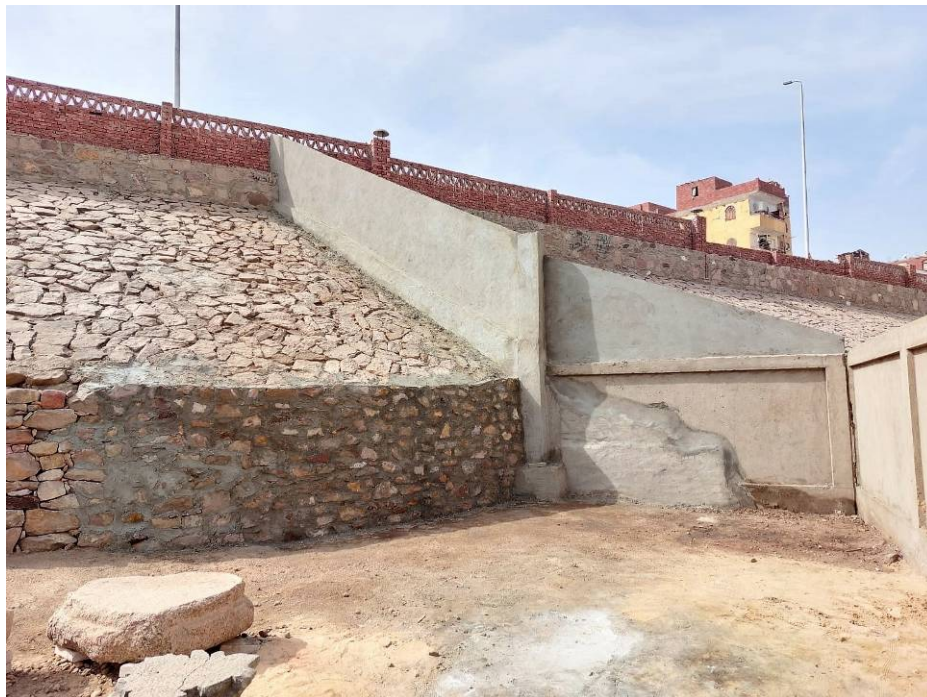
Fig. 3: Area 2: New perimeter wall in the north.
